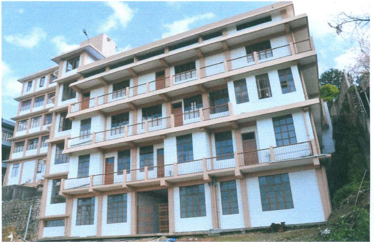
Rear view of the building
